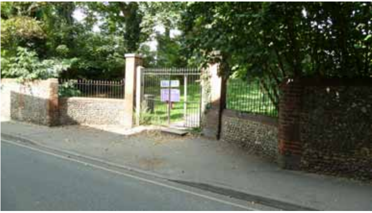
External view of gate, existing
