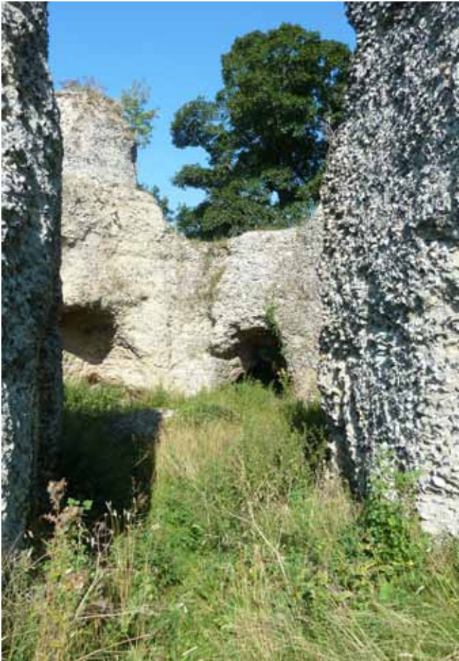
Existing view of Castle interior
